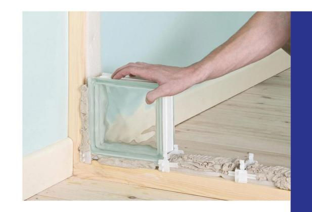
How to use: the minimum and maximum application of each layer is 1 and 5 mm
